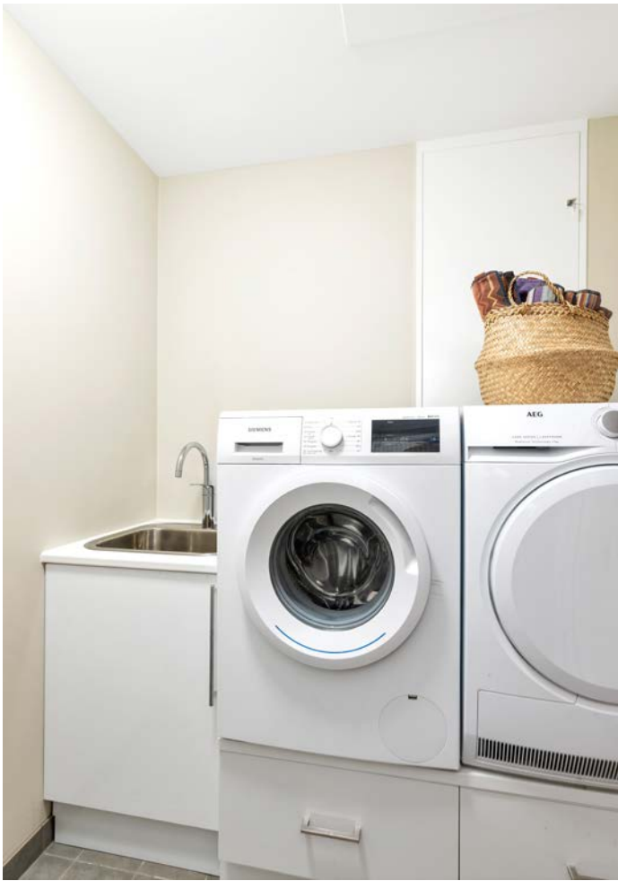
Opplegg for vaskemaskin
