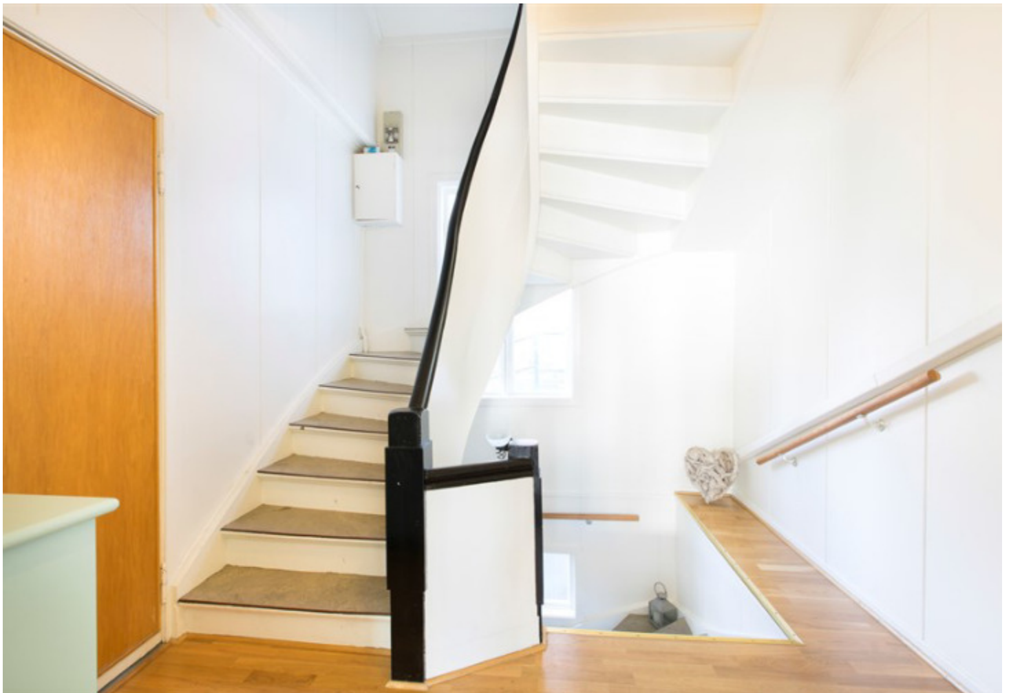
Original trapp i hallen.
