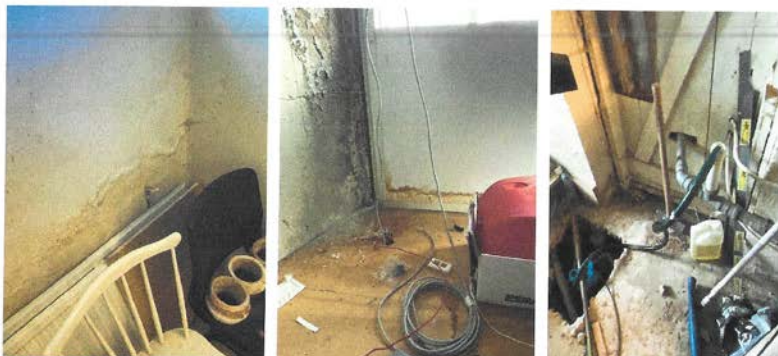
Hull i gulv i bod for pumpe.
