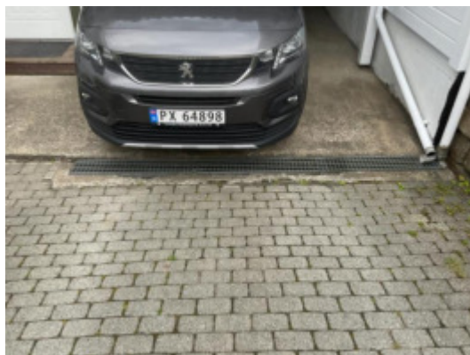
Rist foran carporten.
